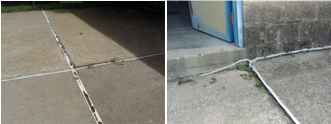
The trench drain is in a state of disrepair and broken but is not seen as vital to the pool's operation. Doors to the locker rooms are in need of some repair.
