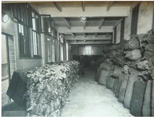
Warehouse of skins around 1930 (Rivet-Chauvard collection)
